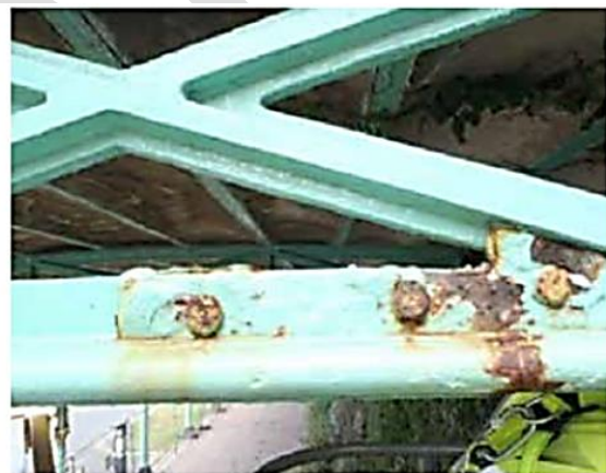
typical bottom chord
