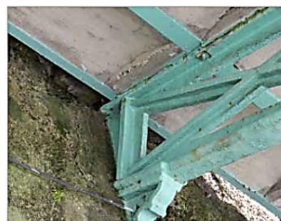
jack arch to lattice beam connection
