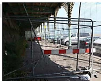
proximity of vehicles to columns
